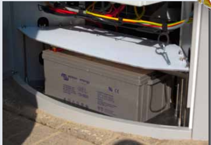
Photo 6 & 7: The Victron batteries and the MultiPlus are fitted in the pillar.
