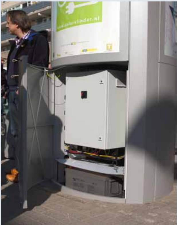
Photo 6 & 7: The Victron batteries and the MultiPlus are fitted in the pillar.
